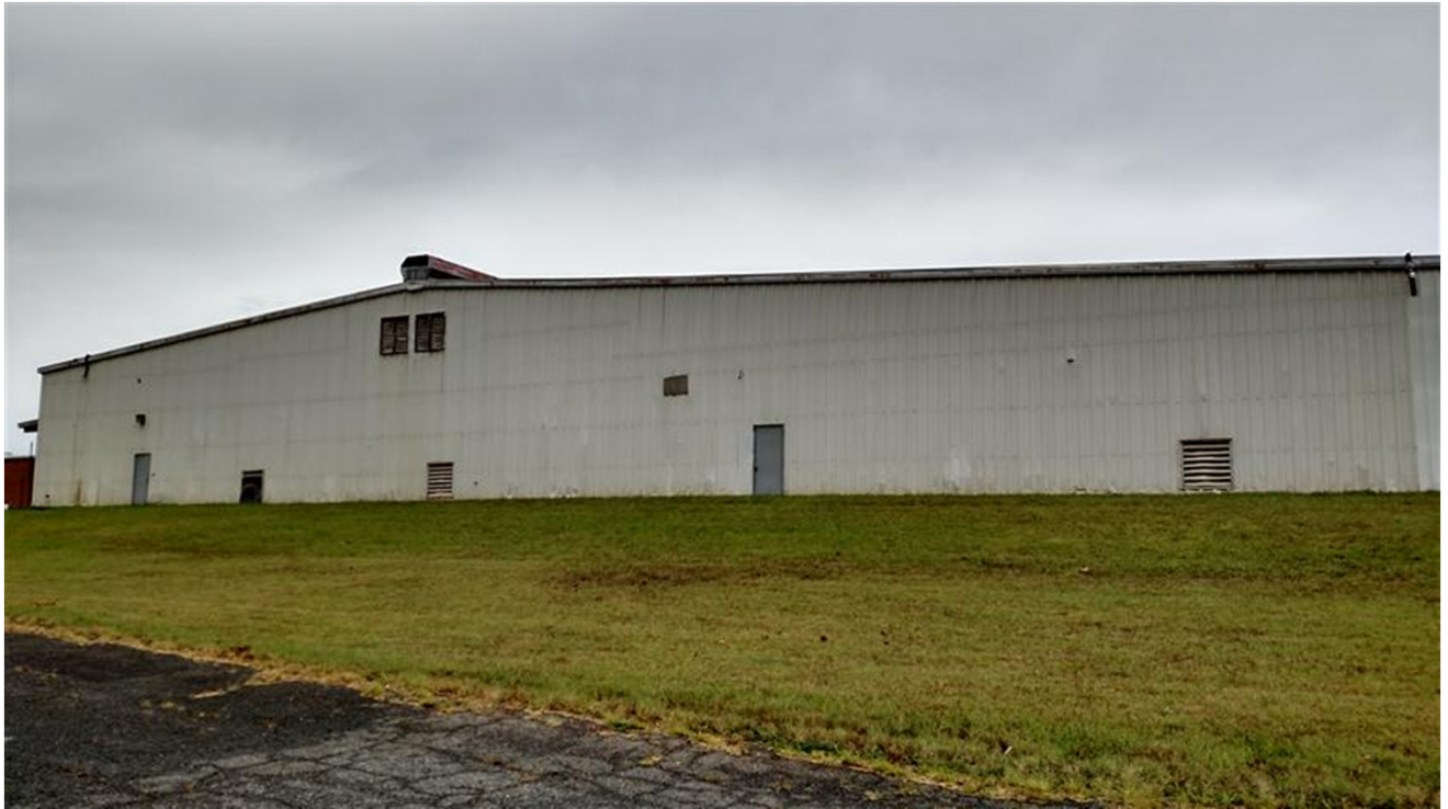
5. Southern exterior wall of the project building.
