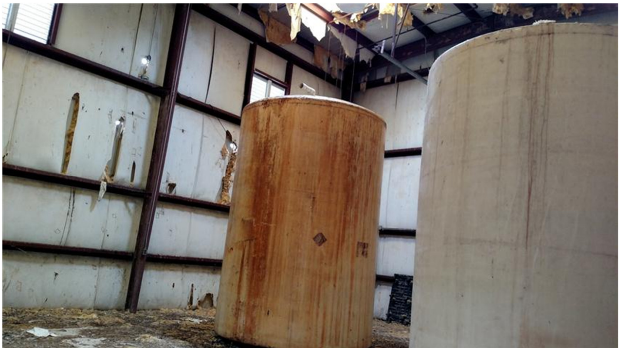
12. Unknown ASTs located in the outbuilding to the south of the project building.
