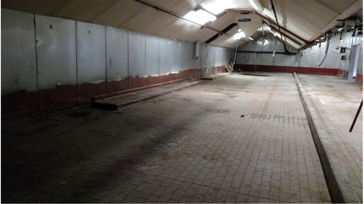
25. Second floor production area
