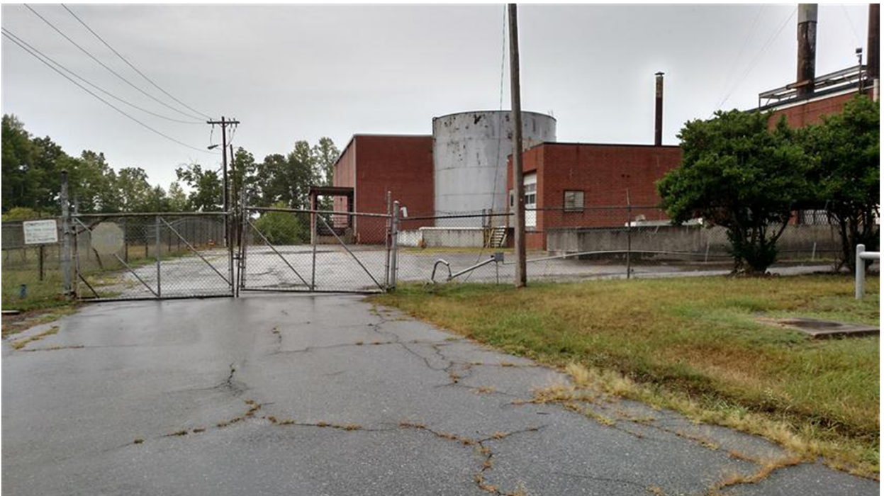
2. View along the eastern exterior wall of the building.
