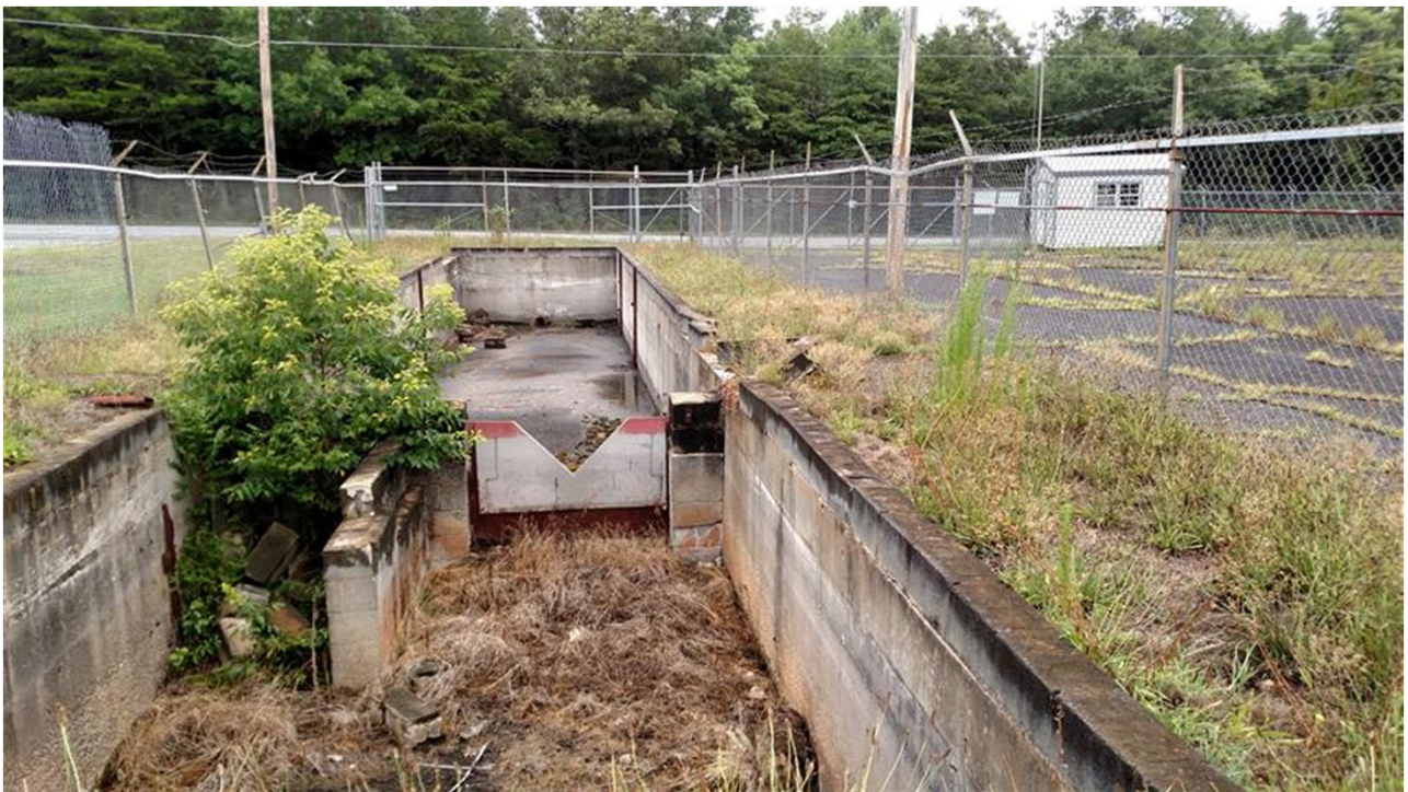
10. View of the effluent sump along the eastern portion of the property.
