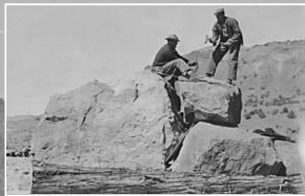
Fastening bolts in "Portal" structure 1936.
