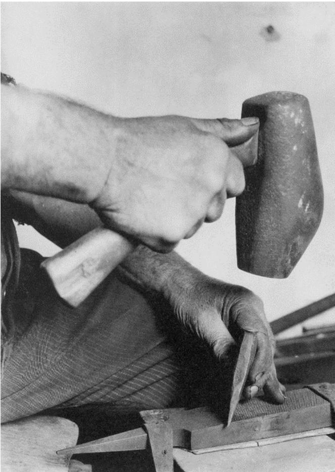
Cutting a file from - Vom alten Handwerk, 1925-1931
