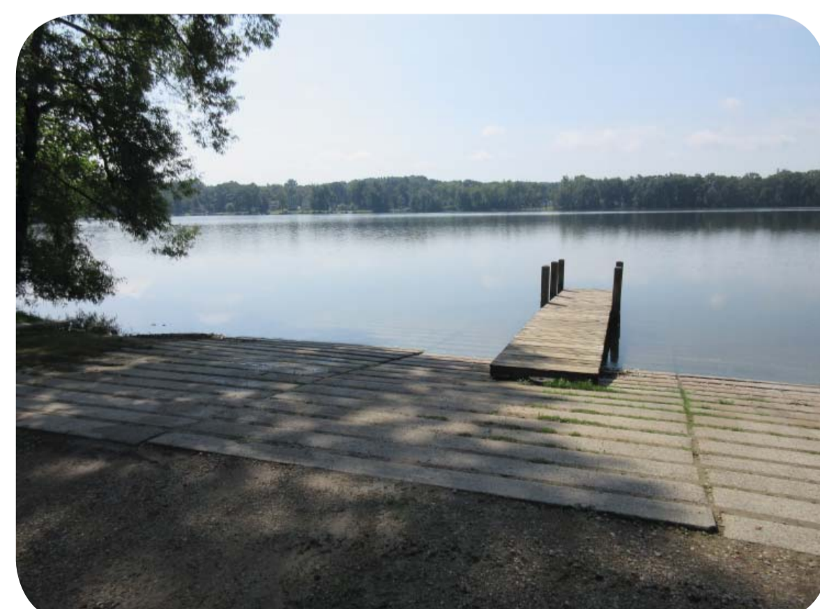
THREE LANE BOAT LAUNCH AREA WITH SKID PIER.
