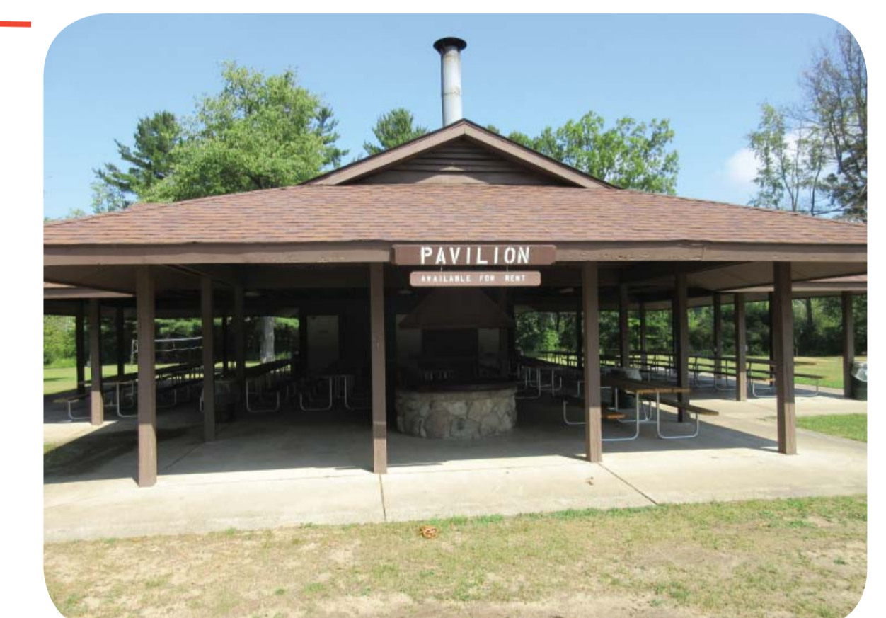
PICNIC SHELTER AND PAVILLION WITH RESTROOMS.
