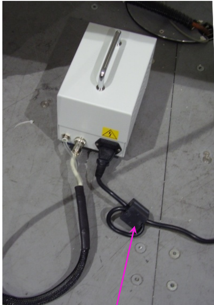
Ferrite bead (with 2 turns) on AC mains cable
