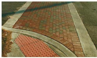
Custom cut bricks used to make curved edges.
