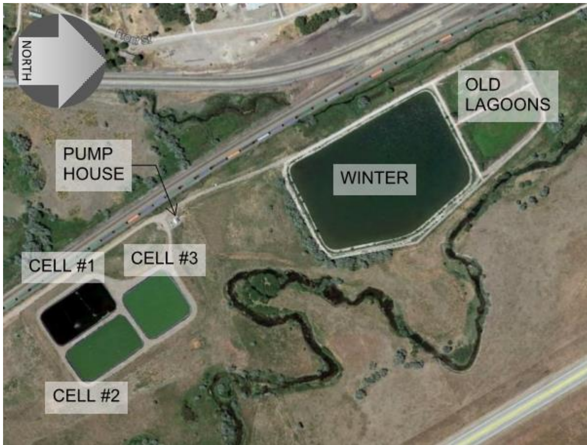
FIGURE 2-2 WWTP AERIAL VIEW
