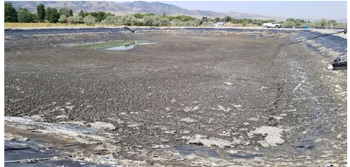
Biosolids accumulation in Cell 1
