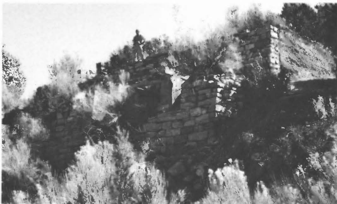
FIGURE 1.7. Foundations of the 100-ton-per-day mill just north of the Virginia mine. Production ceased in 1919.
