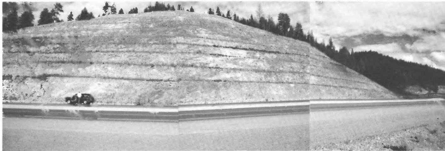
FIGURE 1.31. Panorama of benched, highway-roadcut quarry in San Andres Formation (filled-in karst) at Stop 6, mile 104.5.
