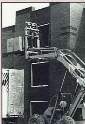
A high loader is used to move desks and beds through the windows of a suite living room. Photo by Kate Johnson.
