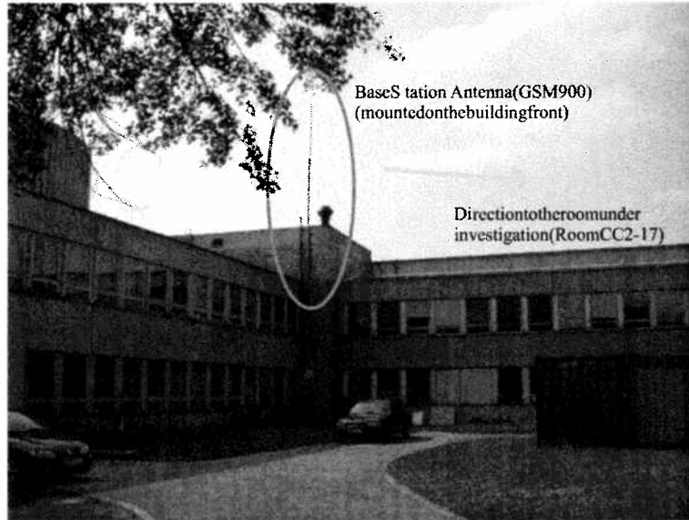
Figure 105: Outside view of the base station antenna mounted on the front of the building (marked with a red cycle) and the direction to the Room CC2-17 which was under investigation.
