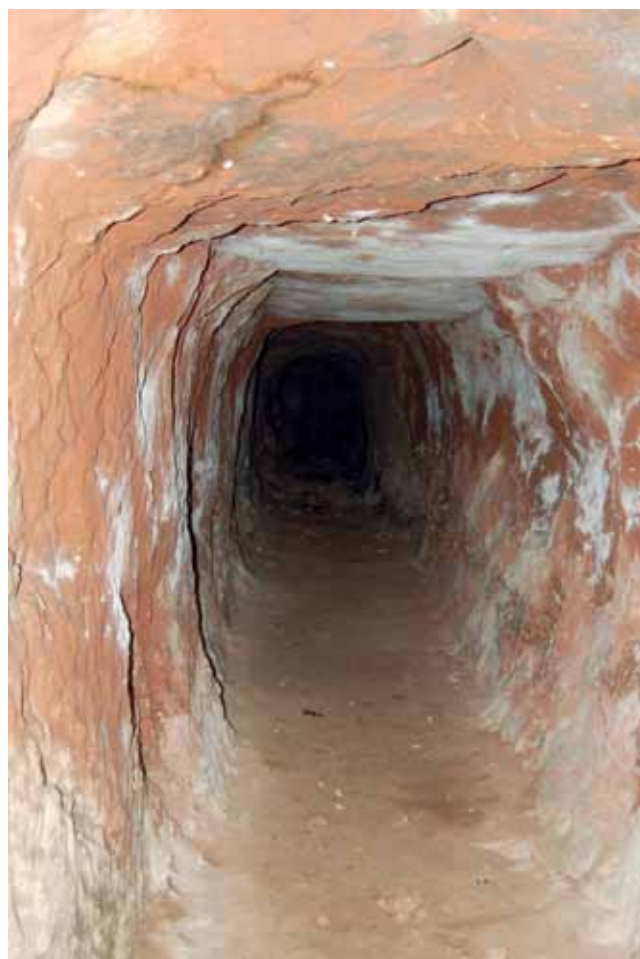
Figure 3. The crosscut entrance level, Pim Hill Mine, looking east. Roy Starkey photograph.
