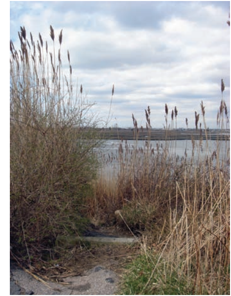
EXISTING COASTAL EROSION CREATED BY RUNOFF FROM ROADWAY
