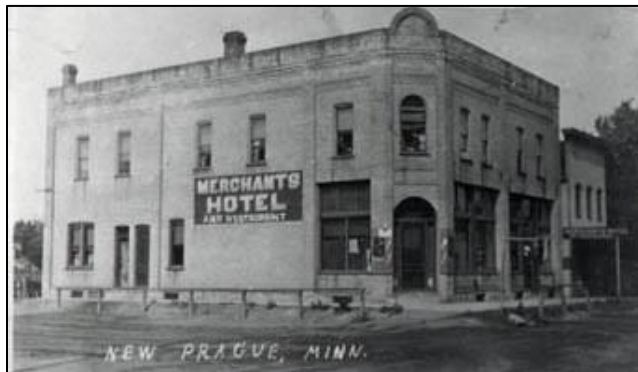
Merchants Hotel – notice the hitching posts located on both sides of the hotel (City of New Prague)
