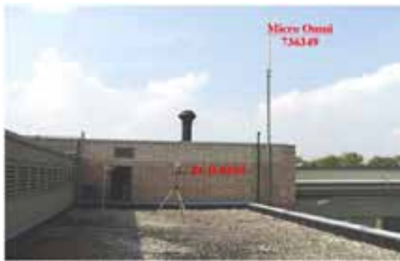
Figure 10: The base station N751 (GSM900) on the rooftop
