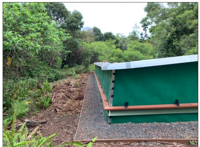
Fig. 4. A recently completed predator-proof fence on Oahu.
