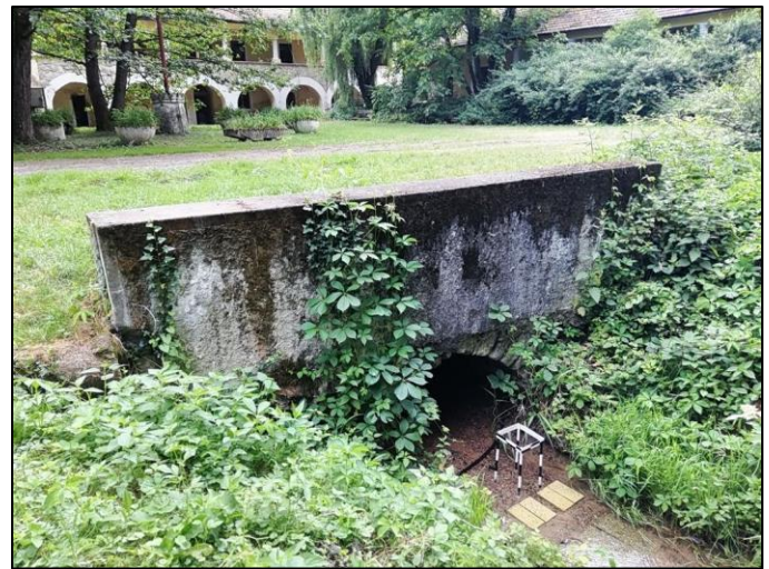
Fig. 4. Test site 1 – tepid-water spring outlet.
