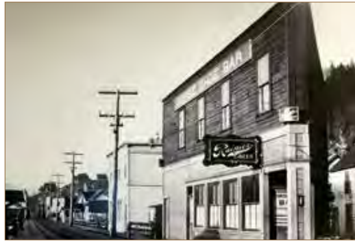
The building at 702 Water St. accommodated Hopkins Way's odd angle in 1912. The sharp vertex was later cut off. Coordination and planning for renewal of Hopkins Alley are under way, aiming to preserve a unique Ketchikan story.
