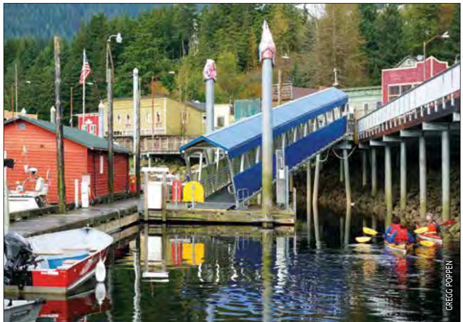
These visitors are paddling near the pilings of a new waterfront promenade and under a new ramp to the Thomas Basin floats. They may not know that they participate in funding this sort of essential infrastructure.
