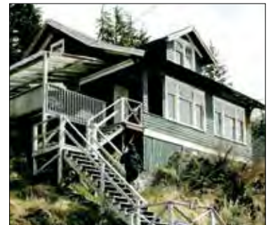
Kubley House (ca. 1917) was built by pioneers whose earlier home was right on the shore of rough-hewn "New Town."
