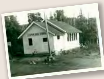
North-end families built Clover Pass School after WWII.
