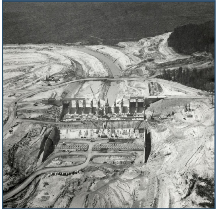
Toledo Bend spillway construction Source: Toledo Bend Lake Country
