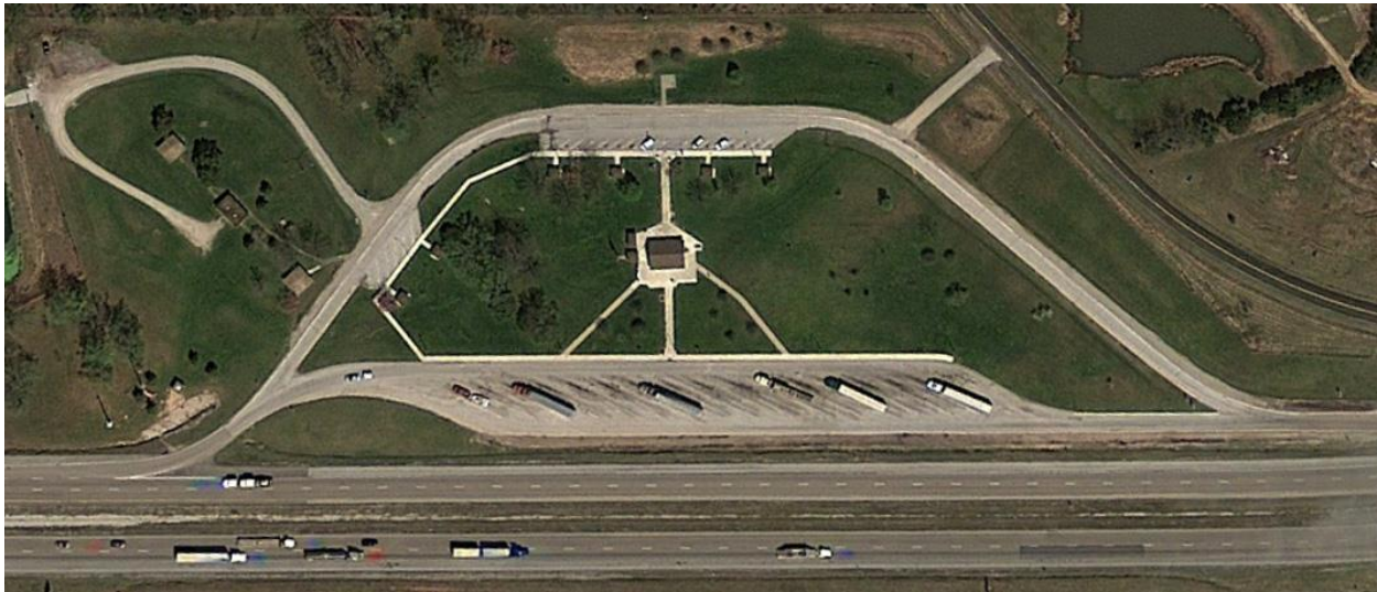
Figure 46. I-70 Rest Area in Danville, Missouri (Before)
