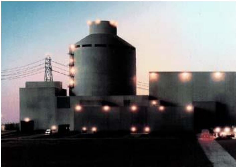
Figure 7. Advanced Passive AP1000 PWR includes a cooling chimney using natural convection in its containment structure. Source: Toshiba-Westinghouse.
