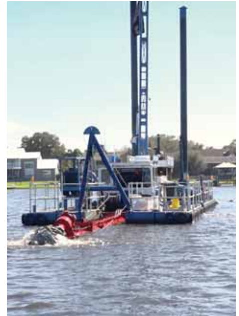
Dredging on Lake Seminole.
