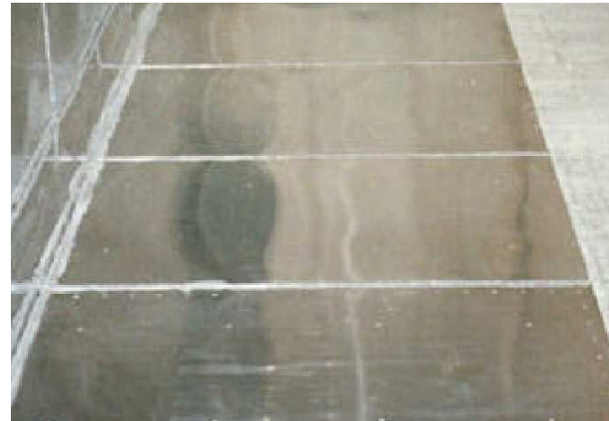
Aaronia Magnoshield® made from Mu-metal allows quick and easy large-area magnetic field screenings.
