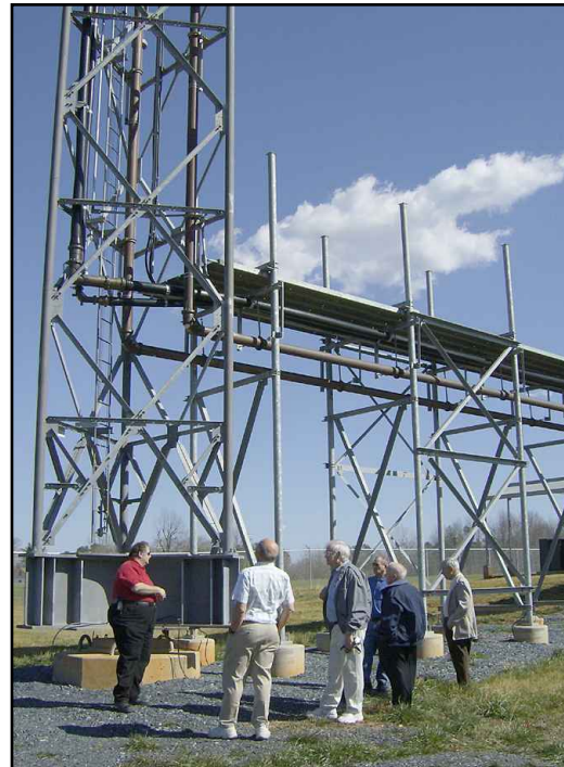
Charles Layno, W4CL, WGHP Fox 8 Transmitter Supervisor, shows the group the new tower base above and in the transmitter room below.
