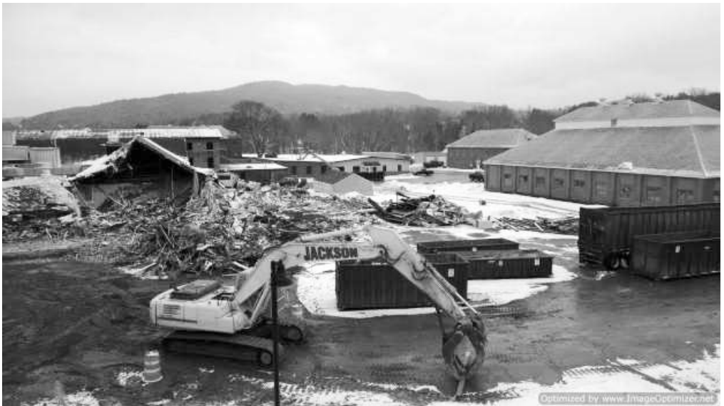
Demolition work on the Old Kitchen at the State Office Complex
