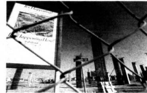
Ballpark construction site
