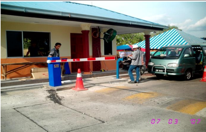
Barrier Gate System – UITM Jengka Phg.
