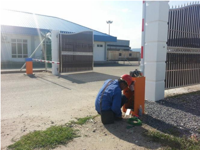
Barrier Gate Installation
