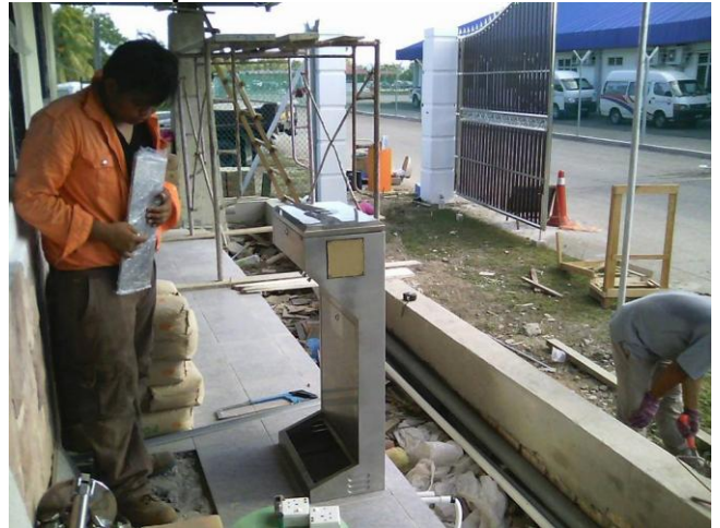
Tripod Turnstile Installation
