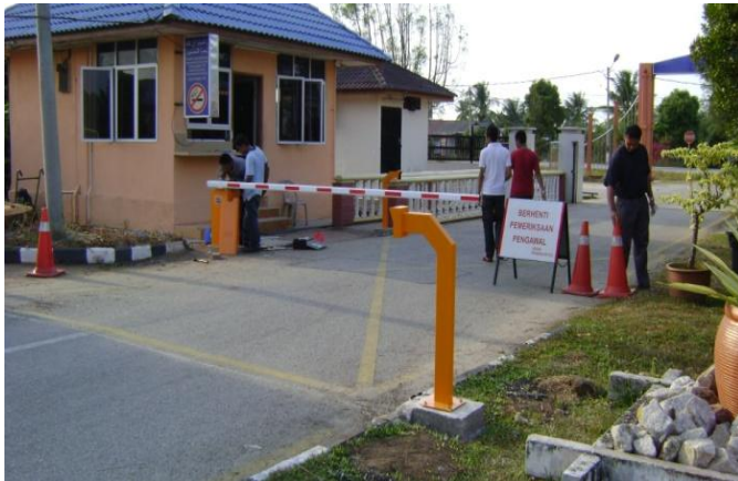
Barrier Gate System – IKM Tasya Pekan Phg.
