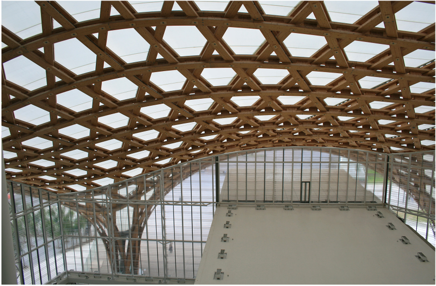
Fig. 4: Wooden structures (such as this one at the Centre Pompidou in Metz, France) store CO 2 over many years.
