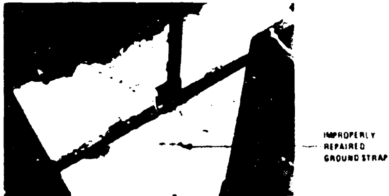
Figure 2-6. Typical Bonding Deficiencies
