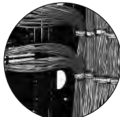
Unique fins support large bundles of cable
