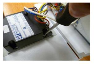
Step 5: Fit new burner controller
