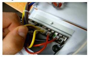
**Step 3:** Disconnect the HT Lead from burner controller.
