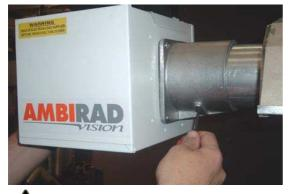
**Step 6:** Remove the burner and position the burner in a safe area to prevent the burner or components attached to the burner from falling to the ground.
