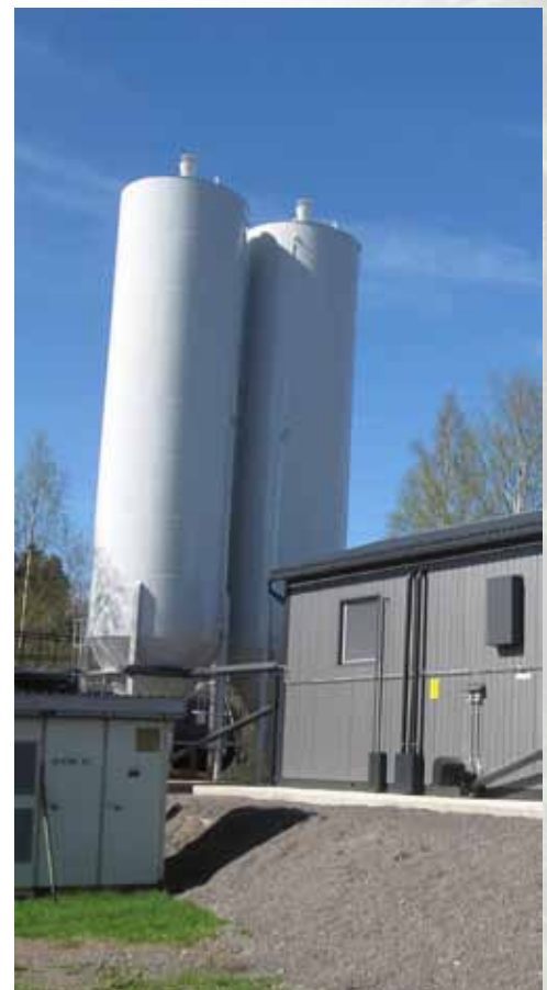
Pellet silos at the heating area of Savon Voima in Sorsakoski
