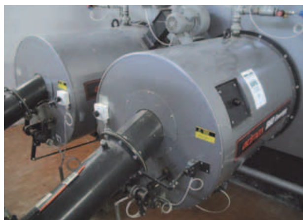
Dual burner solution with BioJet burners.
