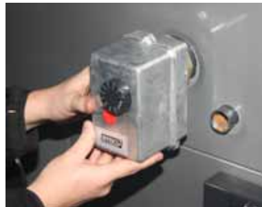
2. Installation of the thermostat
