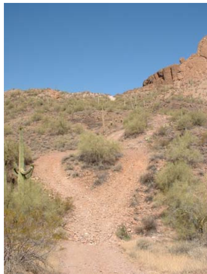
1-15a road splits around Palo Verde severe erosion
