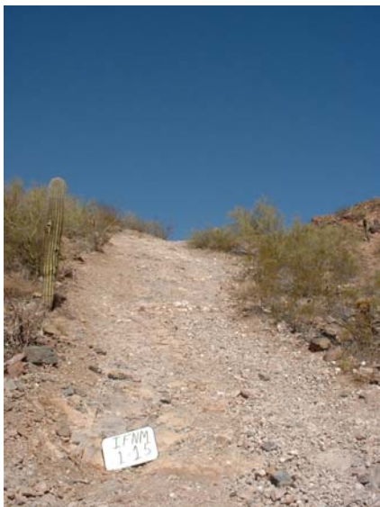
1-15 worst erosion on segment over 15 Degree slope
