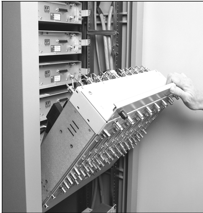
Figure 2-3. Hinge Mount, Side View
