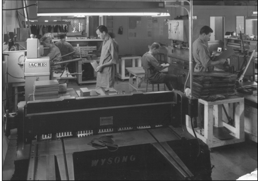
Figure 1-3 Chassis and Cabinet Fabrication
