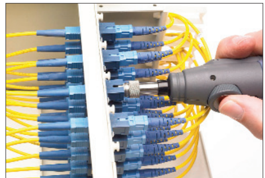
Patch panel bulkhead inspection
