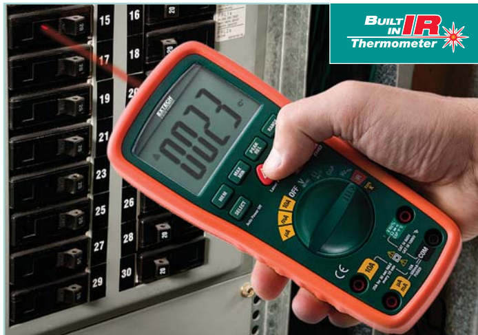
Built-in IR Thermometer quickly identifies hot spots on electrical panels.
