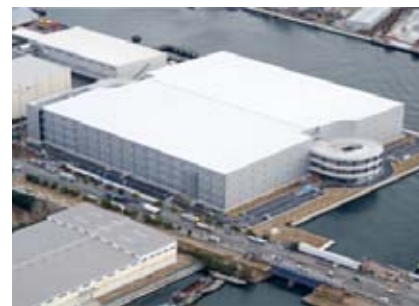
The large, modern Daikoku Logistics Center was completed in March 2010 in Daikoku (Tsurumi Ward, Yokohama). It was developed as a securitized development.
