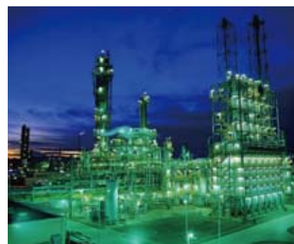
KPI is a joint venture between Indonesian and Japanese companies that can produce 500,000 tons of ammonia a year. It commenced operations in February 2002 as a base for securing basic raw materials for industry.
