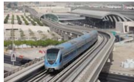
Dubai Metro began operating in September 2009 and is currently used by 100,000 passengers a day. It is quickly becoming an important means of getting about for the citizens of Dubai. MC plans to leverage its experience and success in this project to expand sales of railway systems.
