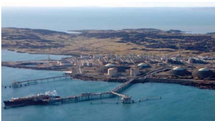
The NWS Project, which began production with two liquefaction trains in 1989, continues to expand. In 2008, a fifth liquefaction train came onstream.
