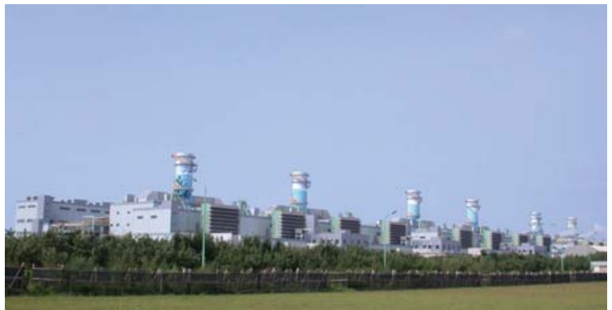
Located in northern Taiwan, the Dah Tarn facility accounts for 21% of the electricity supplied to the region by Taiwan Power Company.
