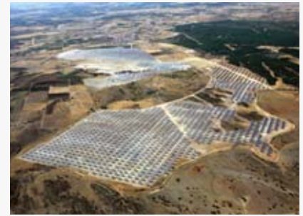
A solar photovoltaic project in Moura, Portugal. Approximately 260,000 solar cell panels are laid out across a site of roughly 250 hectares.
