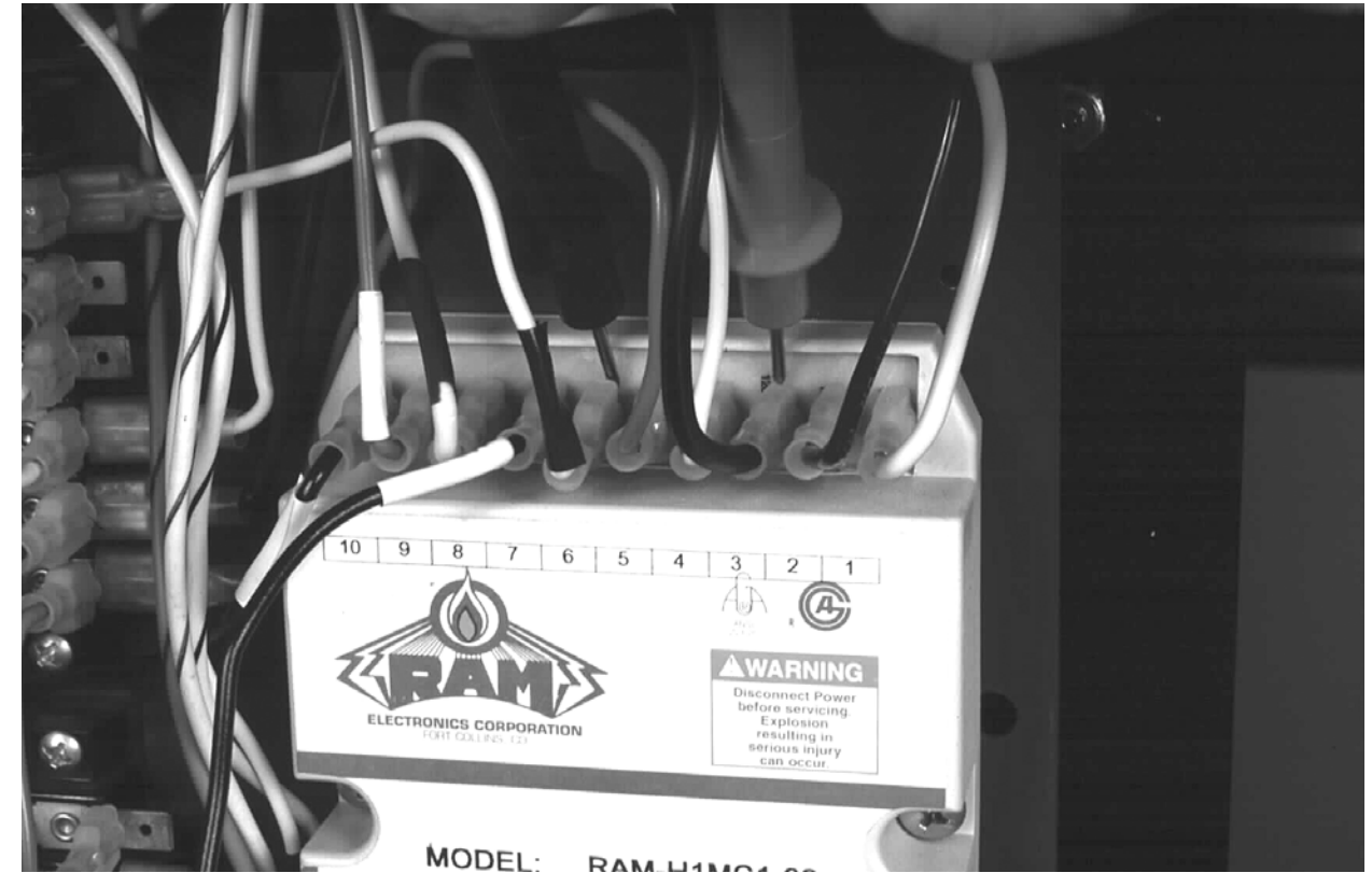
Hot Surface Ignition Control
