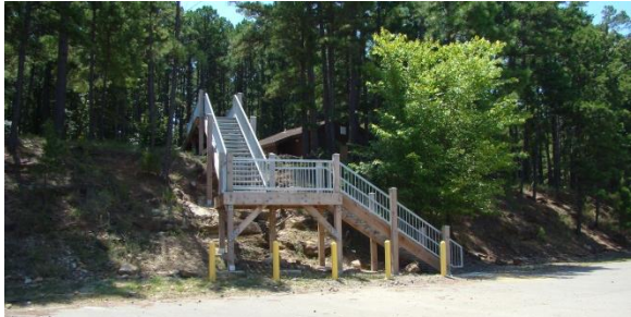
Figure 3.28 – Stairway to comfort station
