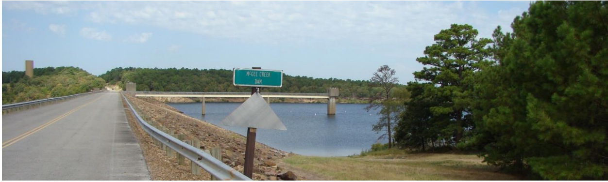
Figure 2.4 – McGee Creek dam
