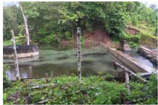
d) Check dam
