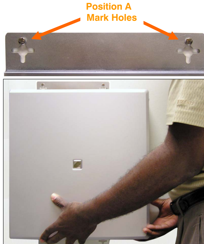
Figure 2.8 Mounting the 7100 Cabinet on the Wall
