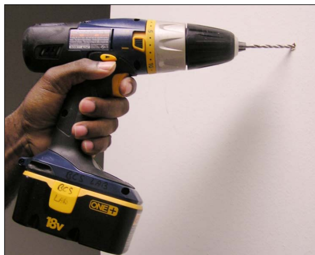
Figure 2.9 Making Holes for Top and Bottom Brackets
