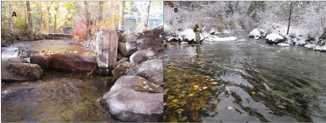
Figure 20. Two of the four pools in Reach 1: A) Small pool downstream of Irrigation out-take weir and related boulder spur at RM. 0.27 (10/24/2017); B) Pool downstream of hillslope contributed boulders at RM 0.39 (11/9/2017).
