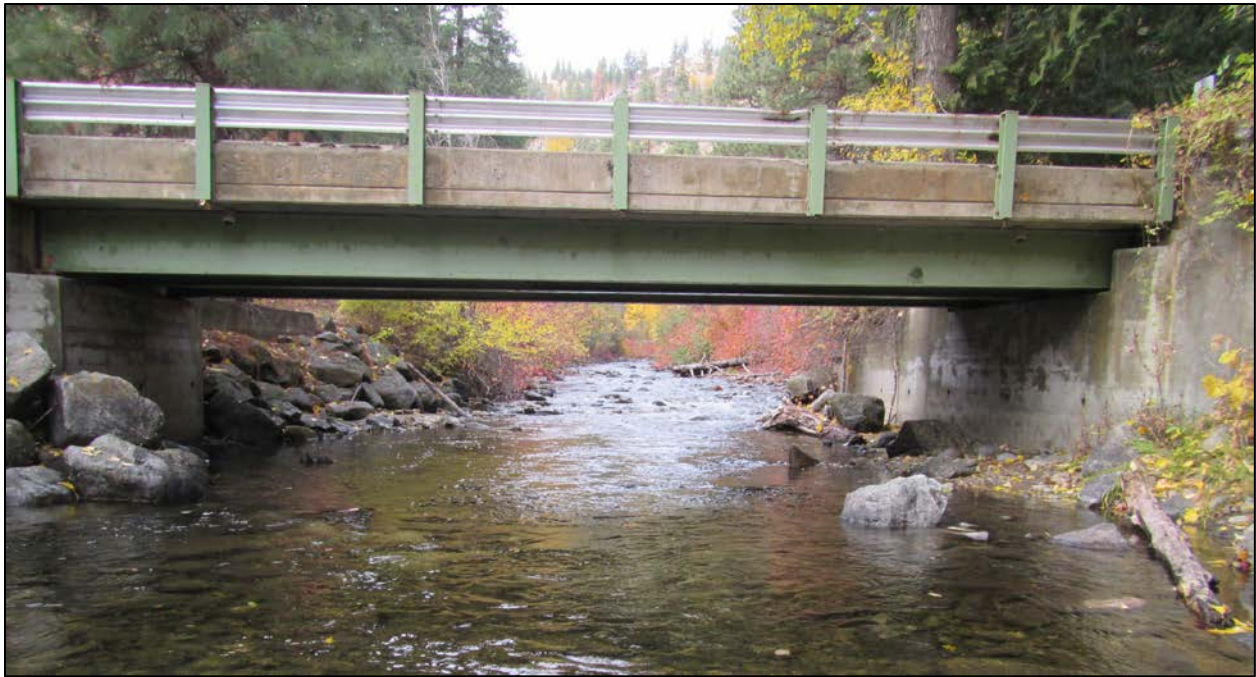
Figure 45. Tillicum Road bridge crossing at RM 2.04, looking upstream. (Photo: IFI 11/25/2017)
