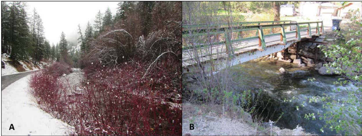
Figure 34. A) Mad River Road along Reach 2 occupying \frac{1}{2} of valley floor at RM 1.55 (Photo: IFI 11/9/2017); B) bridge crossing at RM 0.98 (Photos: IFI 4/25/2018).
