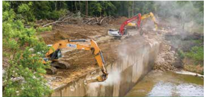
Removal of Green River Lock and Dam #5. Photo: Mike Wilkinson, The Nature Conservancy
