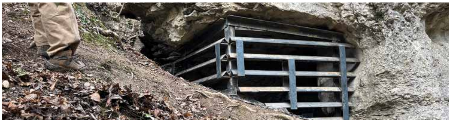
Bat friendly cave gate installed at Virginia big-eared bat maternity site. Photo: Zack Couch
