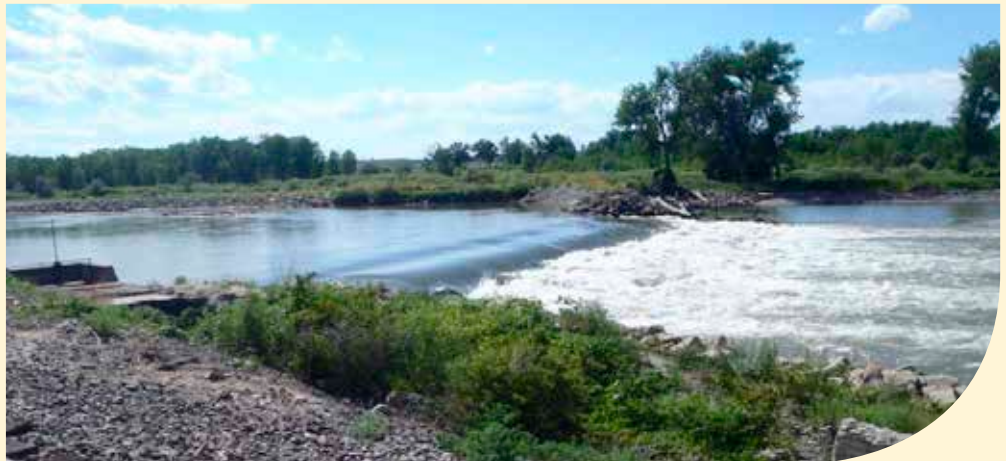
Waco Dam installed on the Yellowstone River.
