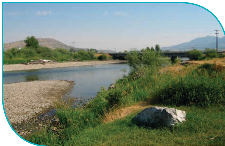
Cardwell Bridge FAS
