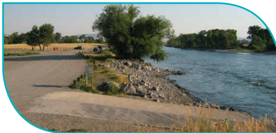
Mayor's Landing FAS
