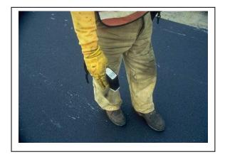
The best way to avoid temperature segregation is with a consistent paving operation. Frequent temperature monitoring, both at the plant and behind the paver, may reveal sources of inconsistencies in mat temperature. Thermal imaging (infrared) cameras are available that can detect temperature gradients in freshly placed HMA. Though not specified in Iowa, some states do require use of infrared cameras to monitor consistency of mat temperature and quickly identify problems as they develop.
