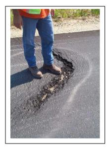
This may require additional rollers or, in some cases, the mixture temperature may be increased slightly to provide more compaction time. Once the mat has cooled below the tender zone, a steel-wheeled roller may be used to finish compaction and remove marks.
