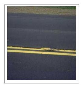
centerline will result in a wide scab of mixture at the surface or the appearance of a white streak at the joint, caused by the roller crushing aggregate in the mix against the surface of the cold mat.
