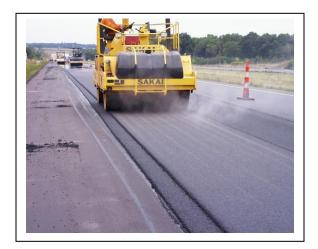
placed. Adjustments can be made to vary the notch depth and wedge slope. A small trailing roller acts to "set" the wedge, while providing some compaction. Conventional methods are used for compaction of the mat itself, and for placing and compacting the second side of the joint (lane) to match.
