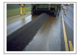
clean and free of moisture before the tack coat is applied. Tack coats shall not be applied when the temperature on the base being covered is less than 25 degrees F.
