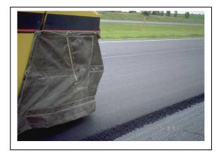
To do so, the roller's spray bars, mats, and scrapers should be in place and properly functioning. Use of approved release agents in the roller's water system may also help prevent mix from sticking to tires and drums.
