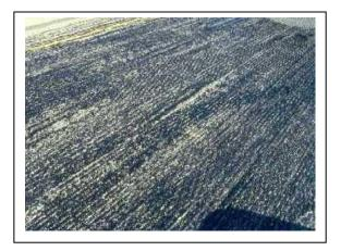
between layers and bleeding of asphalt emulsion to the pavement surface. A pavement that is scarified (milled) requires more tack coat than other surfaces since this process creates more surface area to cover. Rates of application and other requirements for tack coats are given in the contract documents. Tack quantities provided daily by the contractor should be compared with the area covered to verify the rate of application.
