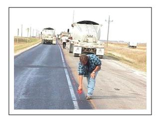
In addition, vibratory breakdown rollers should use <u>low amplitude</u> and <u>high</u> <u>frequency</u> settings to "massage" (rather than "hammer") the mix into place.
