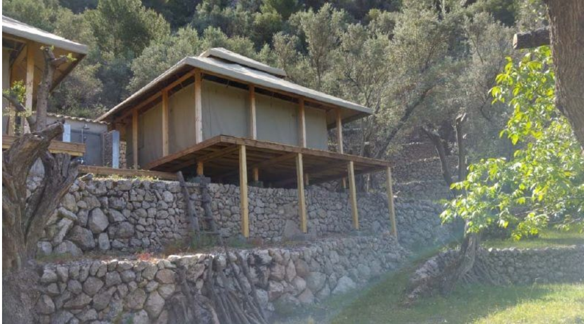
Figure 4.4: One of the two bungalows that, together with a swimming pool, were demolished since they were built without a license in Fornalutx (Serra de Tramuntana), in an area categorised as Natural Site of the Serra de Tramuntana, Natural Areas of Special Interest (ANEI), and Picturesque Landscape.
