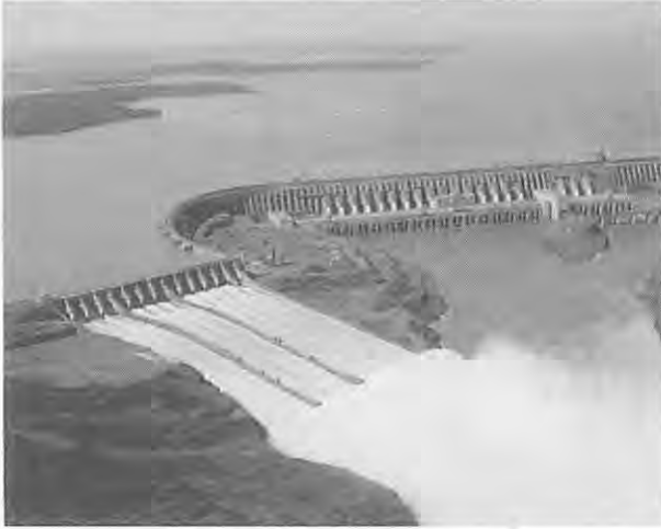
Figure 29-1 The Itaipu hydroelectric dam forming a 200 km-long reservoir (LA: 1347 km 2 ; \bar{z} = 22 m, 12\text{max} = 115m, \bar{x} WRT = 35d) on the Paraná River, on the border of Brazil and Paraguay. The spillway (in operation) prevents flooding of the dam during high water. (Photo courtesy of Itaipu Binacional.)
