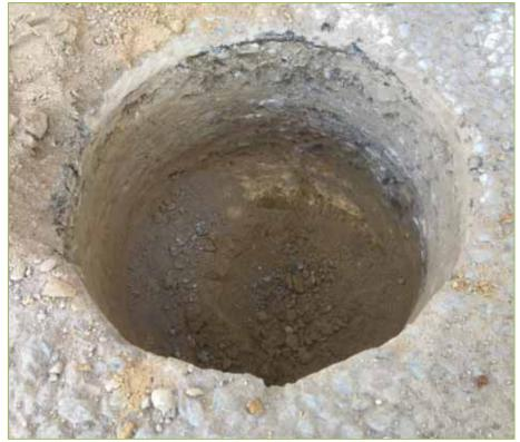
Figure 2.2.11 - BH4: Existing Pavement Structure
