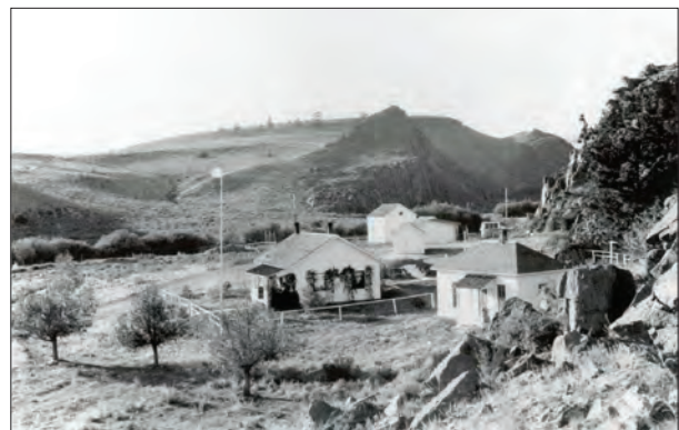
Figure 1.2. Undated photograph of the Upper Saguache Guard Station, probably taken between 1920 and 1938.
