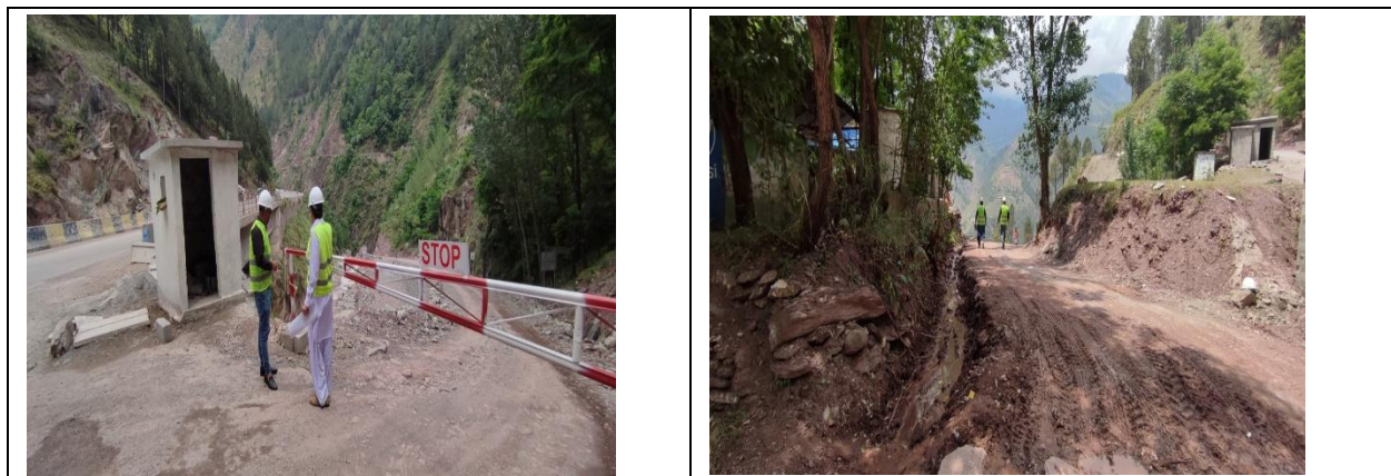
Figure 11: Temporary Access Roads R1 and R3 to access Adits
